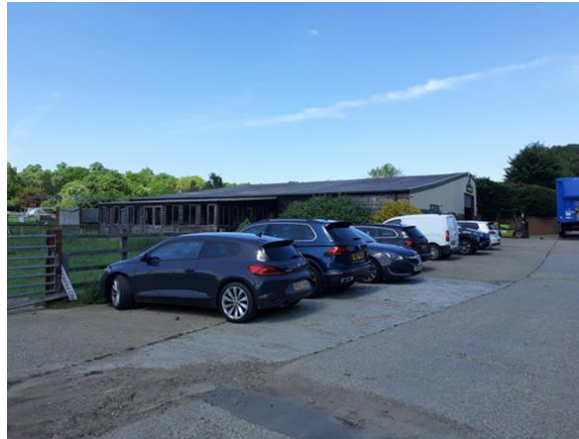
View of agricultural building (side elevation)
