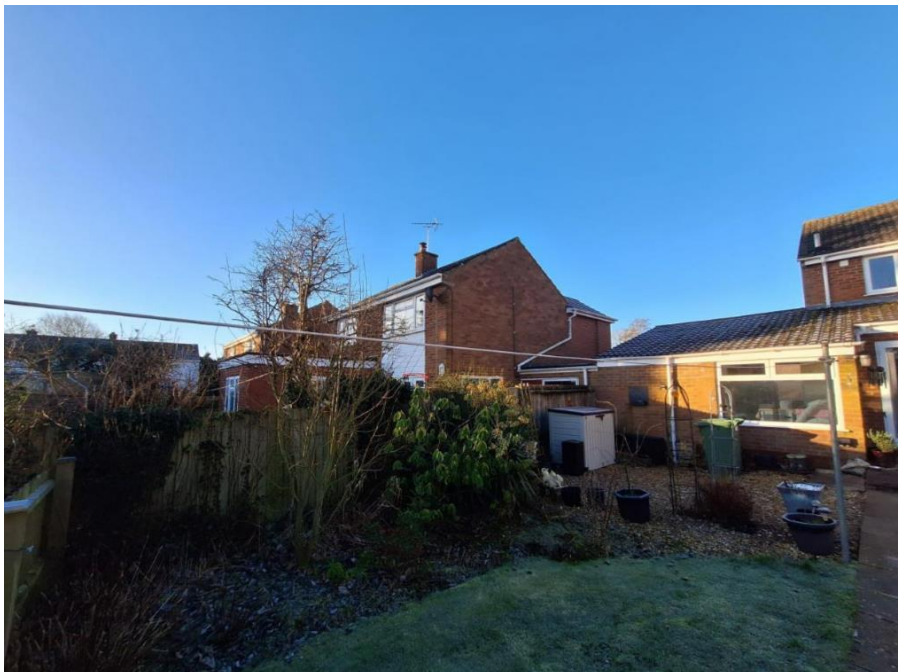
View of No.22 from the garden of No.20
