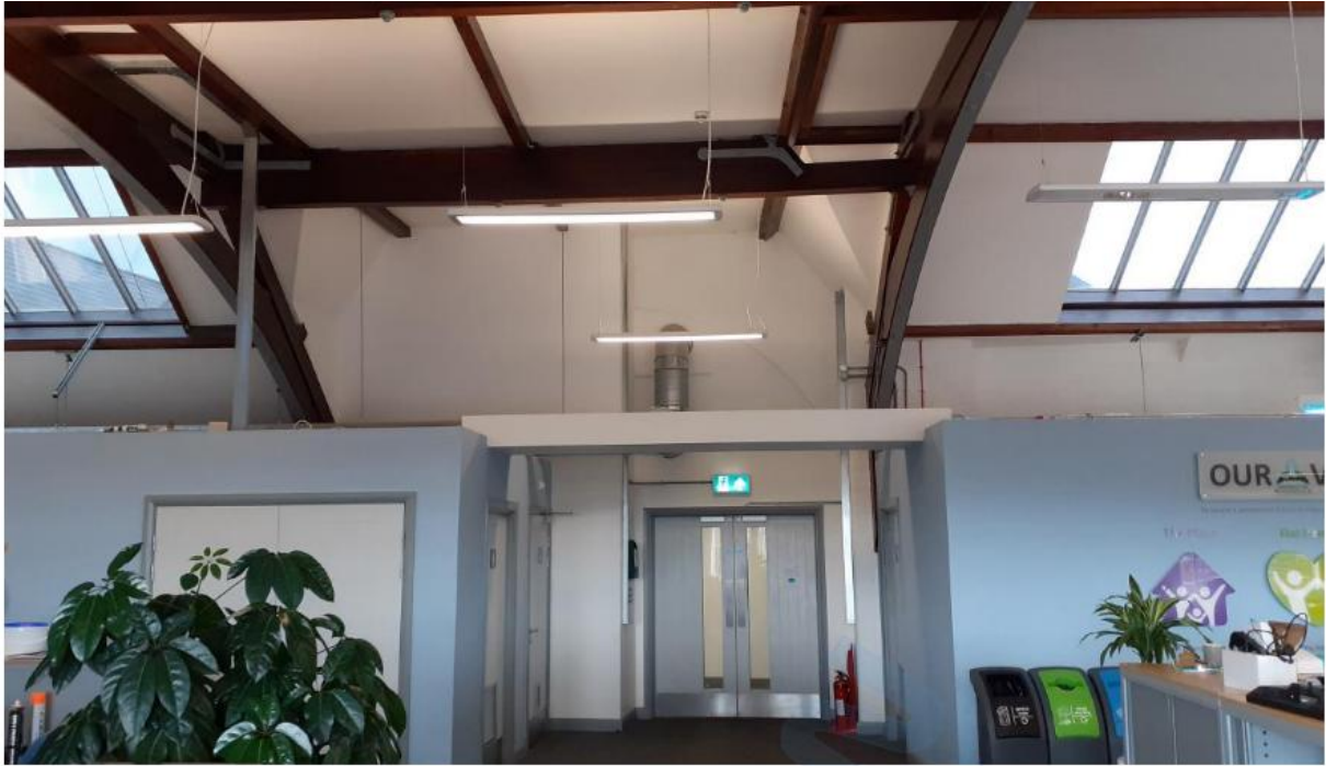
Junction of south range and main stair tower. Existing duct connects WC blocks to 4 th floor plant room
