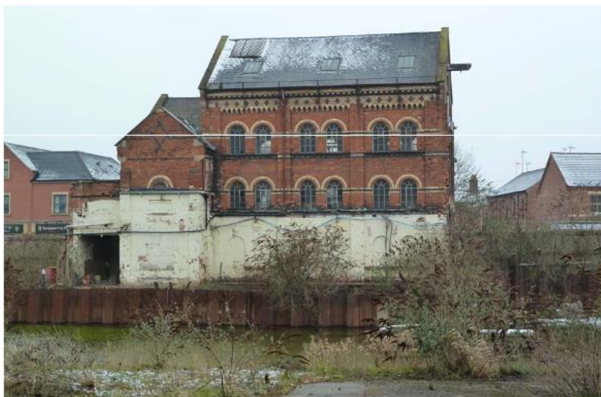
Photo of the southern gable of the Old Flour Mill, clearly showing the line of demolition of a previous factory building. Note all the original ground floor openings have been bricked-in.
