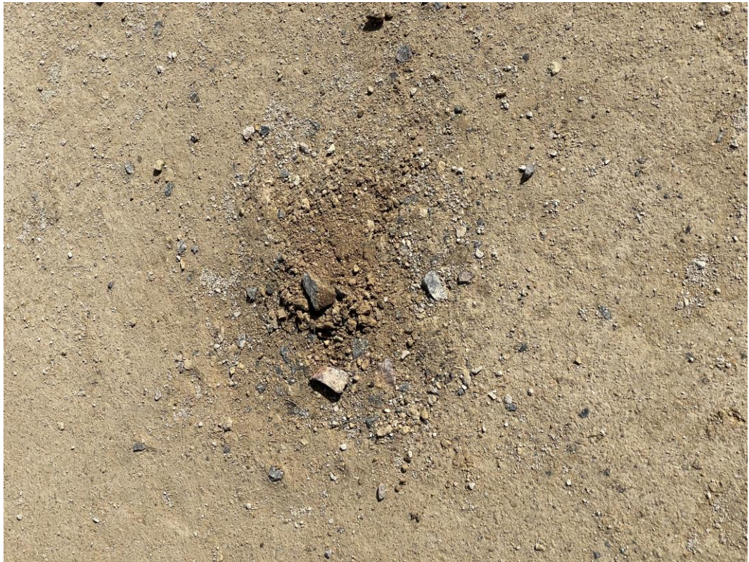
Loose surface material is common with subsurface breaking through creating trip hazards
