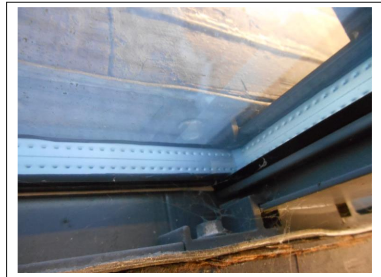
16. Detail View of inside bottom Glazing Unit
