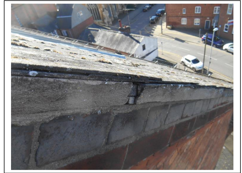
10. Detail View of Undercloak Verge - North Elevation
