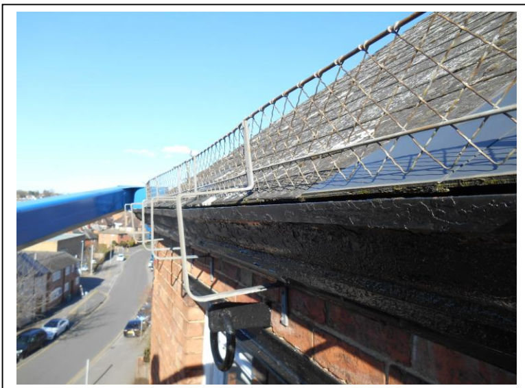
7. General View of Cast Iron gutter/snow guard – East Elevation
