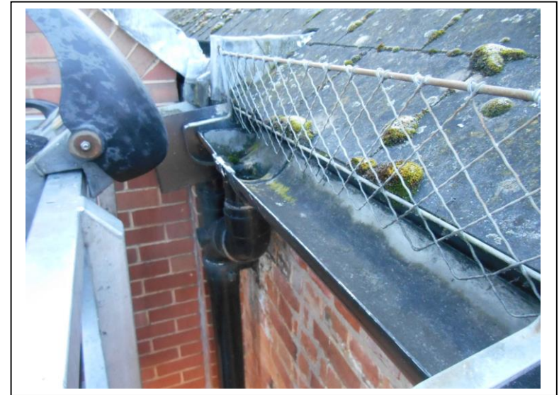
6. General View of PVCu guttering/snow guard – East Elevation
