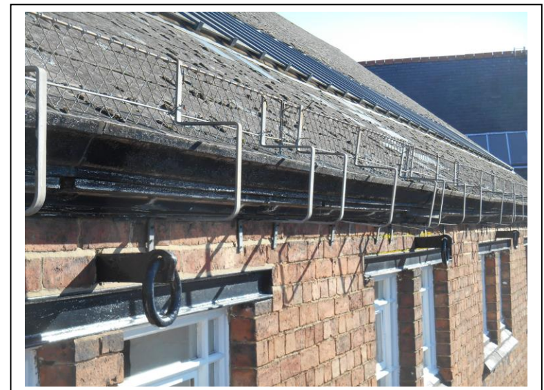
8. General View of Cast Iron gutter/snow guard – East Elevation
