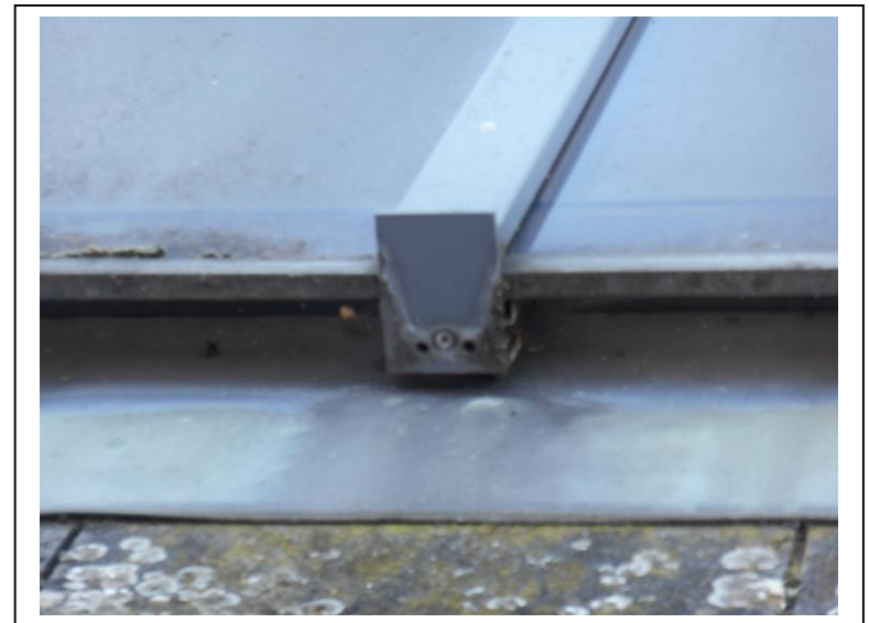
12. Detail View of Bottom edge Strip Glazing
