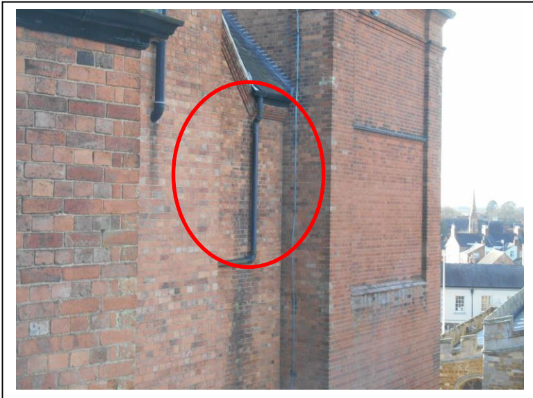
21. View of Rainwater Pipe to replace – Abutment of Rear Wing/Main Building
