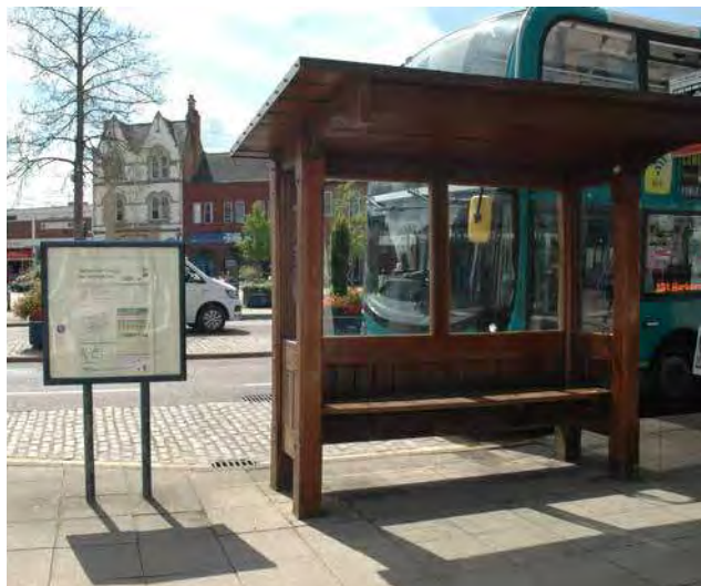
Bus shelter opposite the Square
