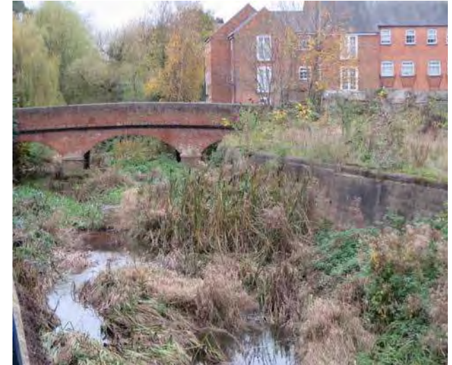
Welland east of Kettering Road bridge
