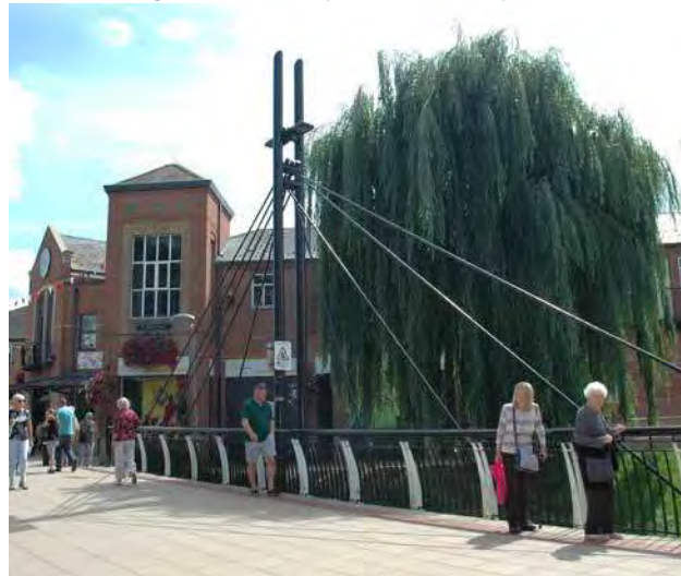
Pedestrian bridge over the River Welland
